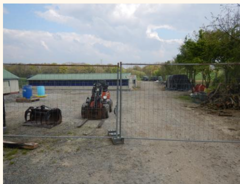
Partial enclosure of the production zone
